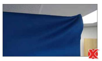
Avoid graphic bunching, especially in the corners which is a problem caused by stretching or pulling the silicone. This occurs most commonly when installation is started at one corner and the edging is 'slid in' along the frame to the other corner, where any excess with gather and look untidy or distorted. For the correct way to get started, check out Tip #3.
